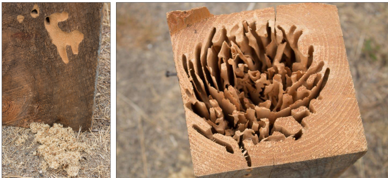
Galleries dug by carpenter ant workers in a barn support beam: view from the outside of the beam (left) and cross-section of the same beam showing the amount of damage within the beam (right). Credits: China Wong, UNH.
