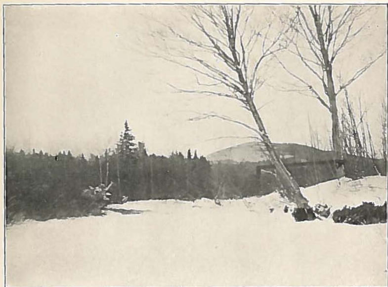
GAGING STATION ON ZEALAND RIVER AT TWIN MOUNTAIN, N. H. Showing conditions on February 10, 1906. Chain gage is on the right. River is frozen over and covered with snow.
