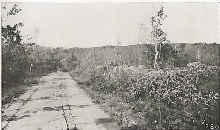
BUSHES CUT AND LEFT ALONG HIGHWAY—A FIRE TRAP.
