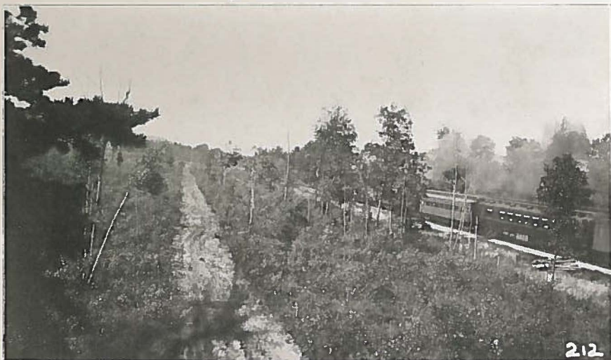
DEBRIS BETWEEN FIRE LINE AND RAILROAD WILL BE BURNED FREQUENTLY. RAILROAD FIRE LINE—MAST YARD STATE FOREST.
