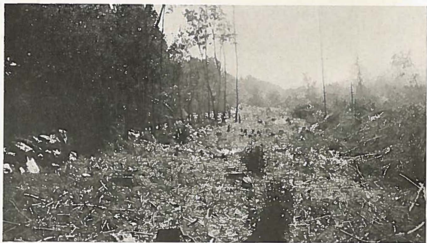
BRUSH CLEARED FROM TWENTY-FIVE FOOT STRIP BESIDE THE HIGHWAY.
