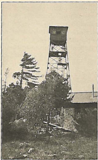
Photo by Forestry Department NEW FIRE LOOKOUT TOWER AND CABIN ON FEDERAL HILL NEAR MILFORD
