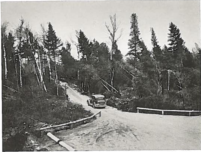
Hazardous blow-down, White Mountain National Forest, before clean-up. (Photo by U. S. Forest Service)
