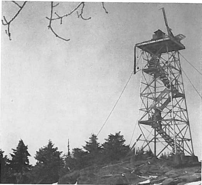
Miller Park tower cab destroyed by lightning February 1960. When enlarged cab was built, no steel was used above floor.
