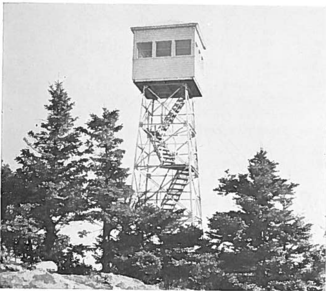
Rebuilt cab in 1960 with lightning protection. Standard practice is to evacuate towers during lightning storms. Cabins have lightning protection.
