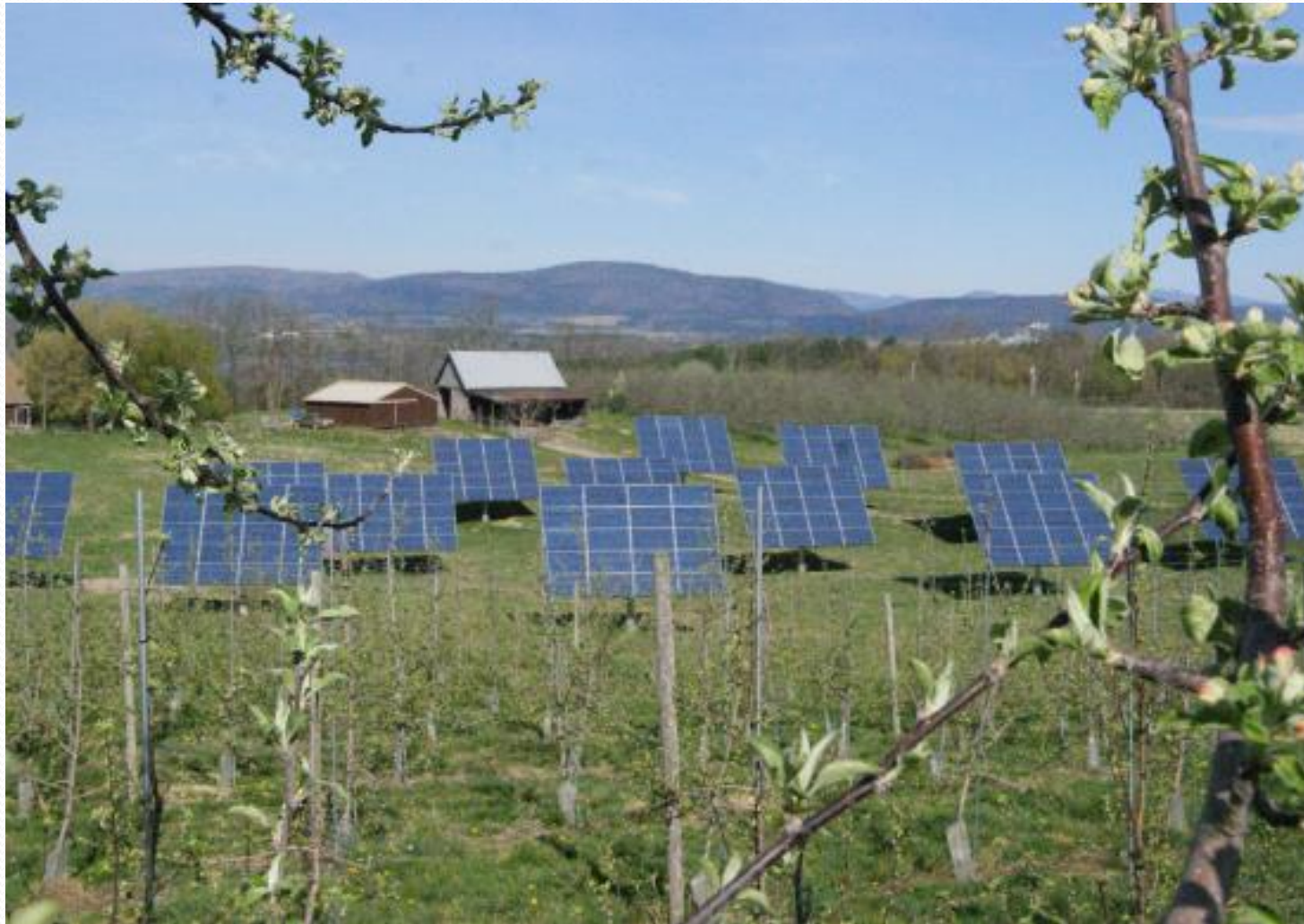
Two 60 kW solar tracker arrays power the processing and value-added equipment at an apple orchard in Shoreham
