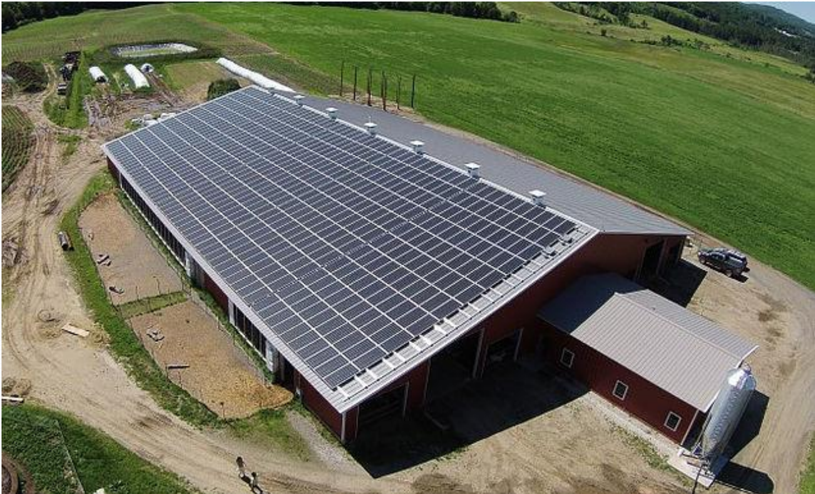
181 kW roof top solar array on goat barn at Ayers Brook Goat Dairy in Randolph
