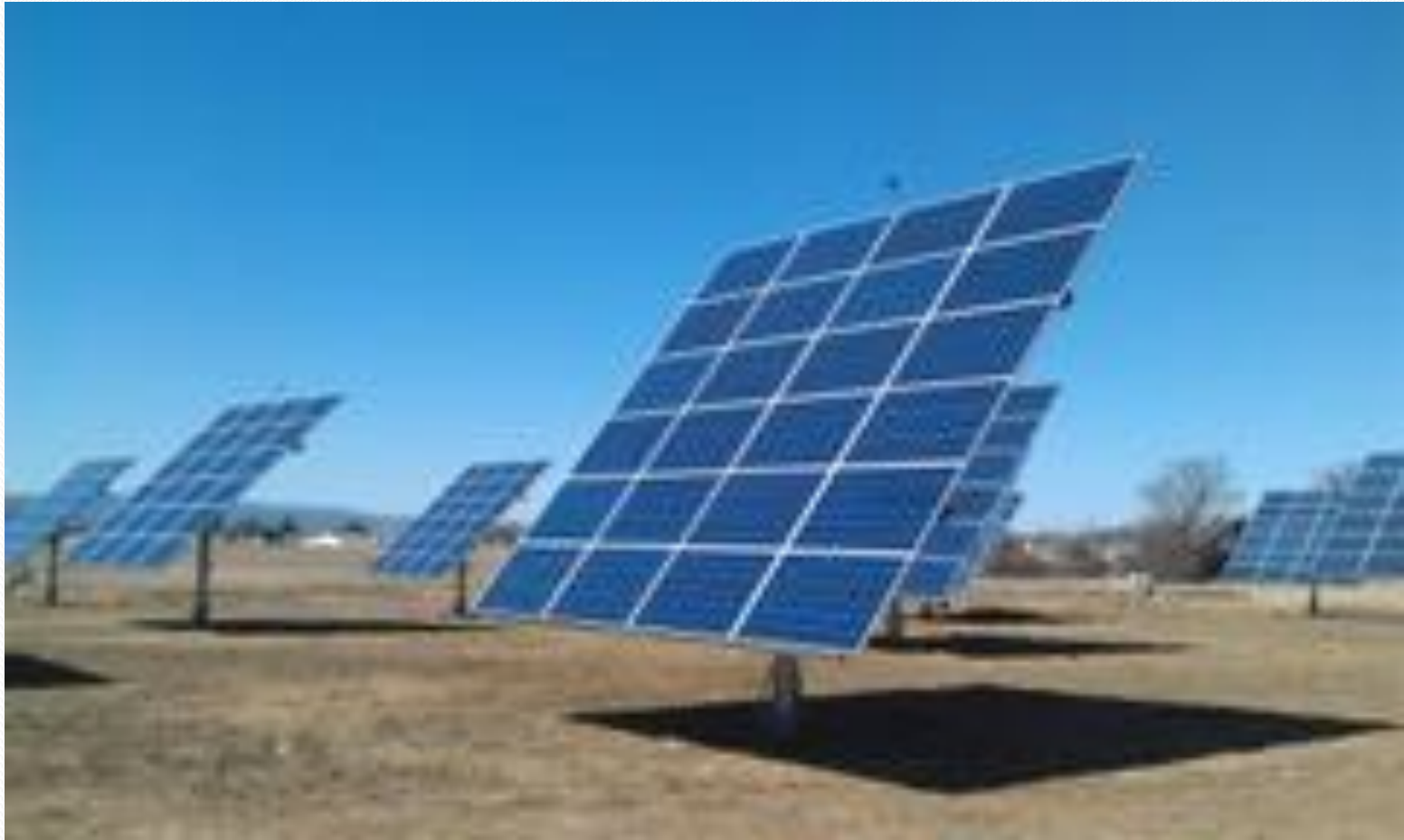
150 kW solar array on land owned by the Town of Williston powers municipal buildings and street lights
