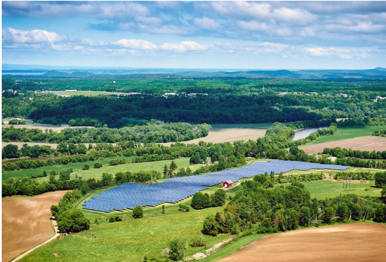
3.6 MW Solar array on land excluded from conservation on dairy farm in Essex
