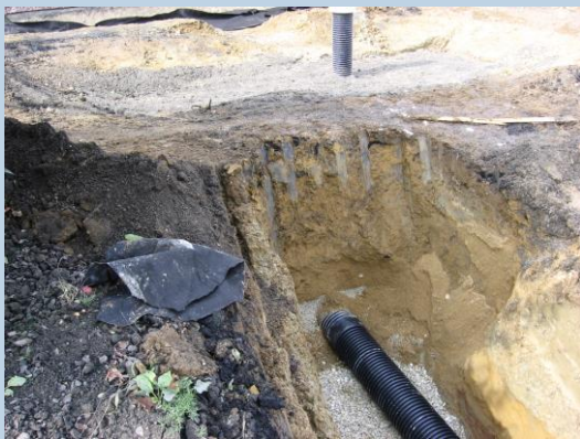
Photograph 5: Hillcrest Avenue infiltration trench.
