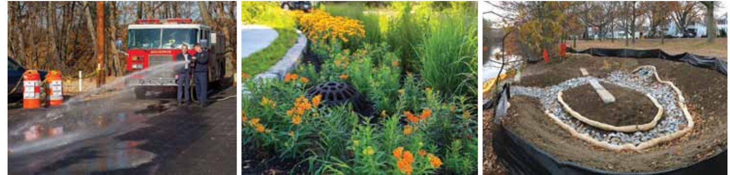
Alongside infiltration trenches, Arlington has employed other small-scale stormwater control systems, including (left to right) porous pavement, rain gardens, and updated outfalls
