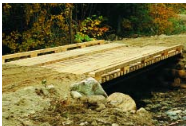
A permanent bridge.
