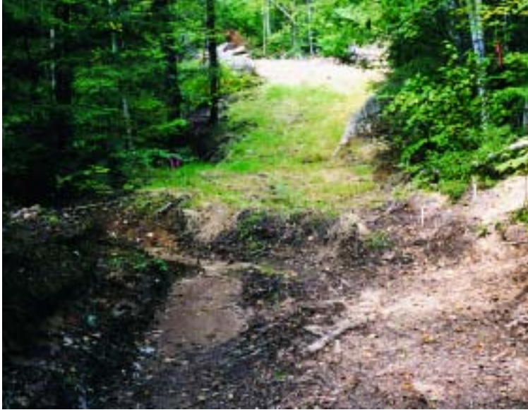
A trail closed-out with water bar and seeding.
