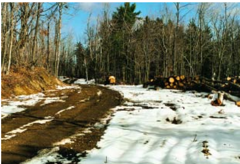
A well-maintained, well-drained landing.
