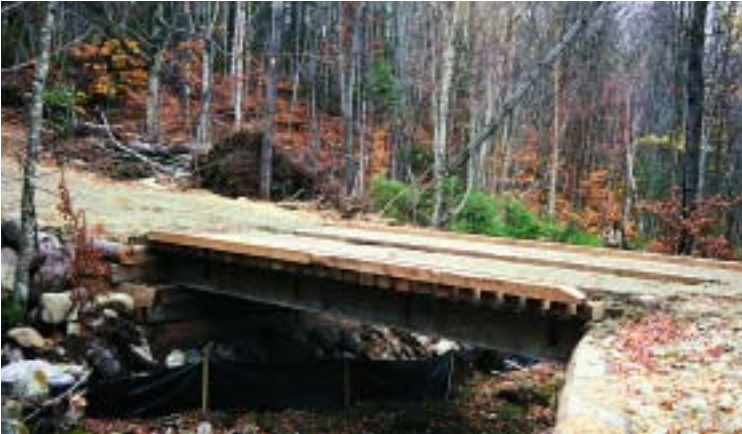
A permanent bridge on a truck road.
