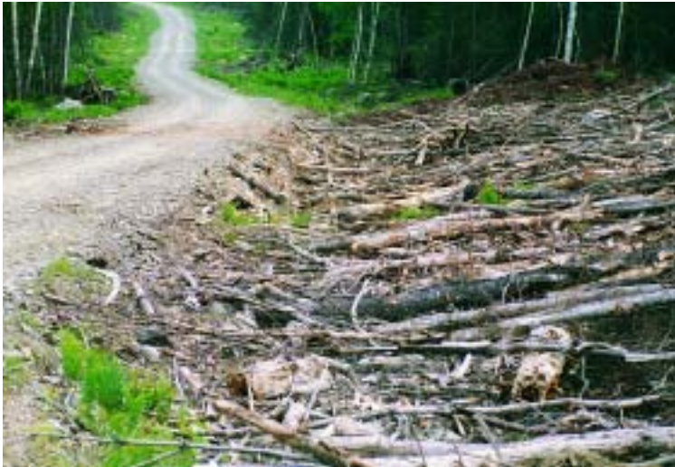
Slash and logging debris can help stabilize exposed soil on log landings.
