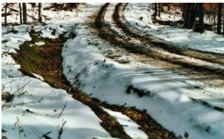
Properly sized ditches capture and slow down runoff.
