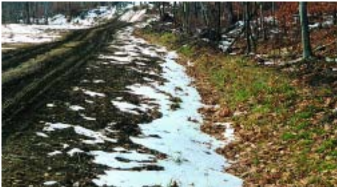
Revegetated road ditches carry water without eroding.
