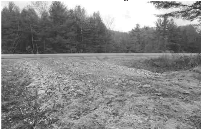
A crushed stone and gravel apron onto NH Route 11 in Wilmot. Photo by H. Johnson, NHTOA
