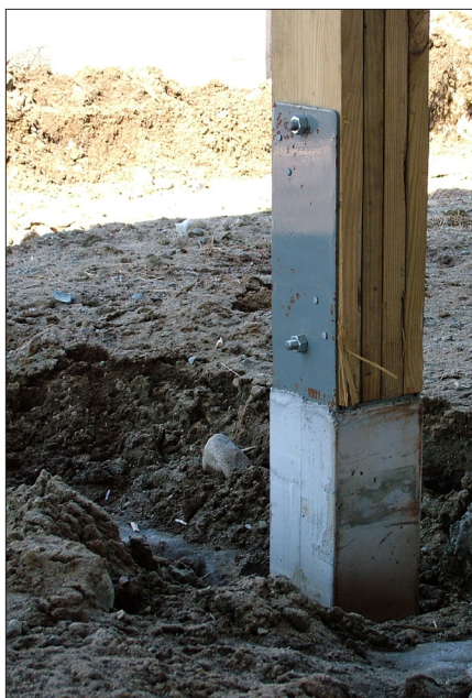
Laminated post on a pre-cast concrete base.
