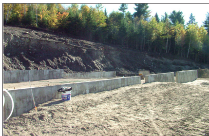
Spend time removing the topsoil at the site and add a gravel base larger than the building to promote flow away from the structure.
