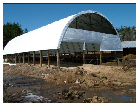
The hoop structure provides a lot of flexibility for uses with animal housing. The top part of each end should be covered with shade cloth to provide ventilation. Side “pony walls” can provide a space for curtains and protect the roof material from animal damage.
