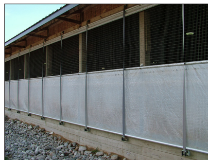
Adjustable sidewall curtains can replace enclosed walls and provide ventilation.
