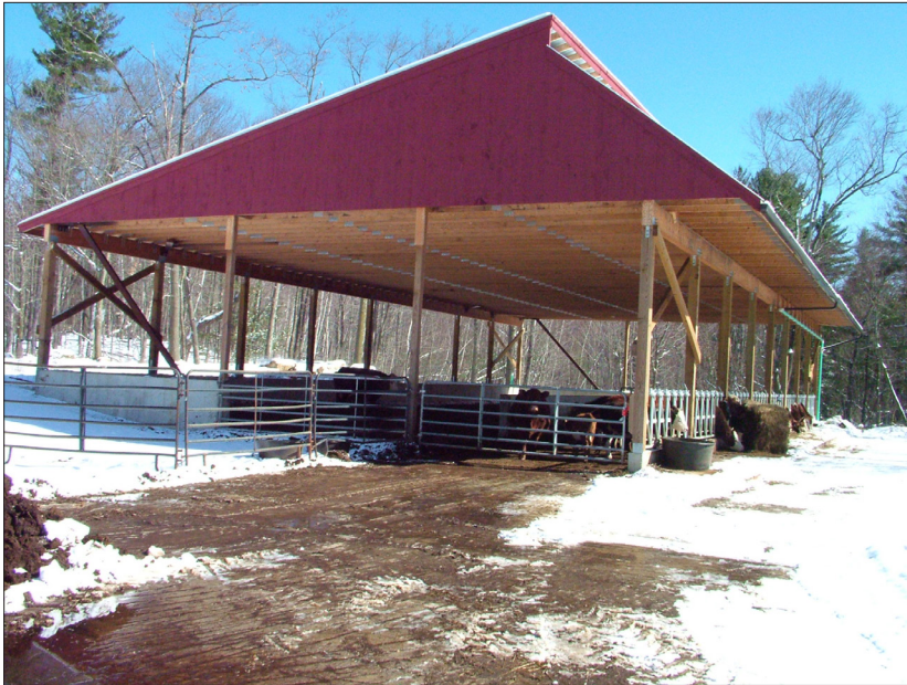
A pole barn with clear-span trusses is a good building option for many farms.
