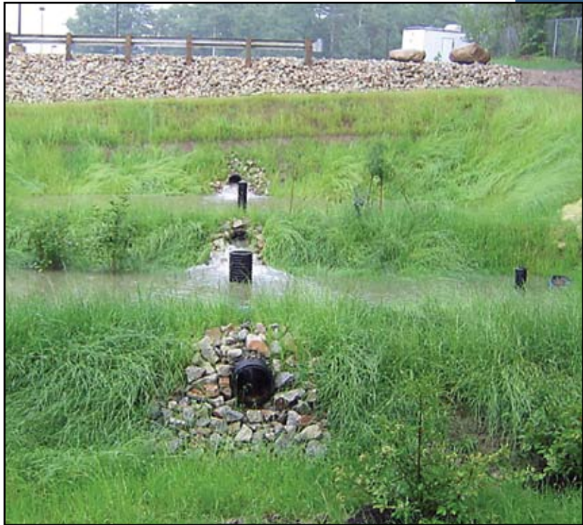
Gravel wetland operation in a rain event.
