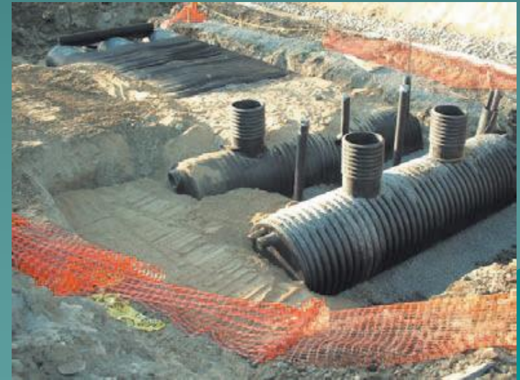
ADS Infiltration System
