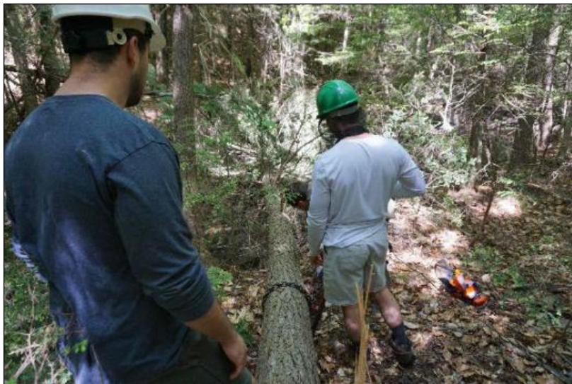
Field technicians Luca Trotta & Drew Dunlap setting up the grip hoist to move a felled tree into position.
