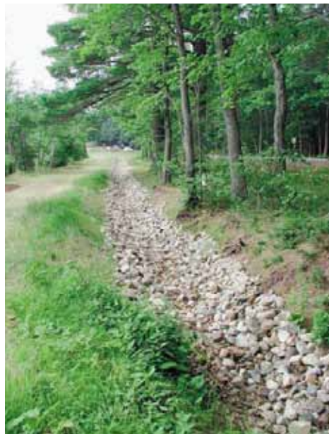
A swale constructed along this roadway captures road runoff and prevents it from entering the lake, which is to the left.
